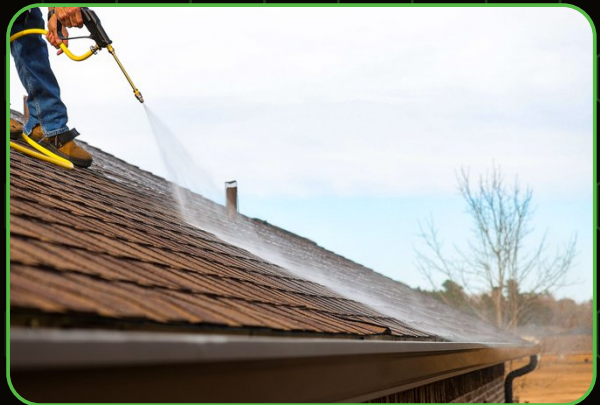
Ridge-to-eave application workflow.
