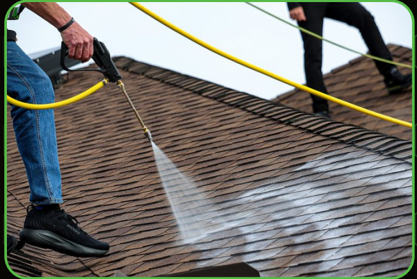
Even, low-pressure spray coverage.
